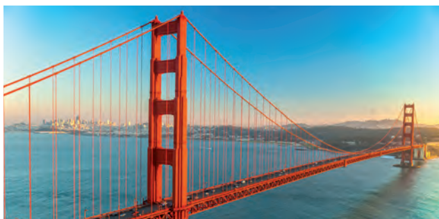
Figure 1: The bridge that CAN needs to reach the US is not finished yet
